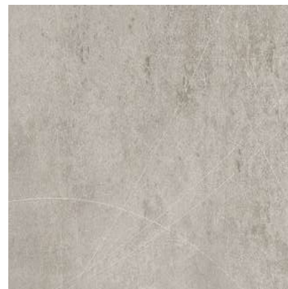
NOT-3994 Scratched Concrete
