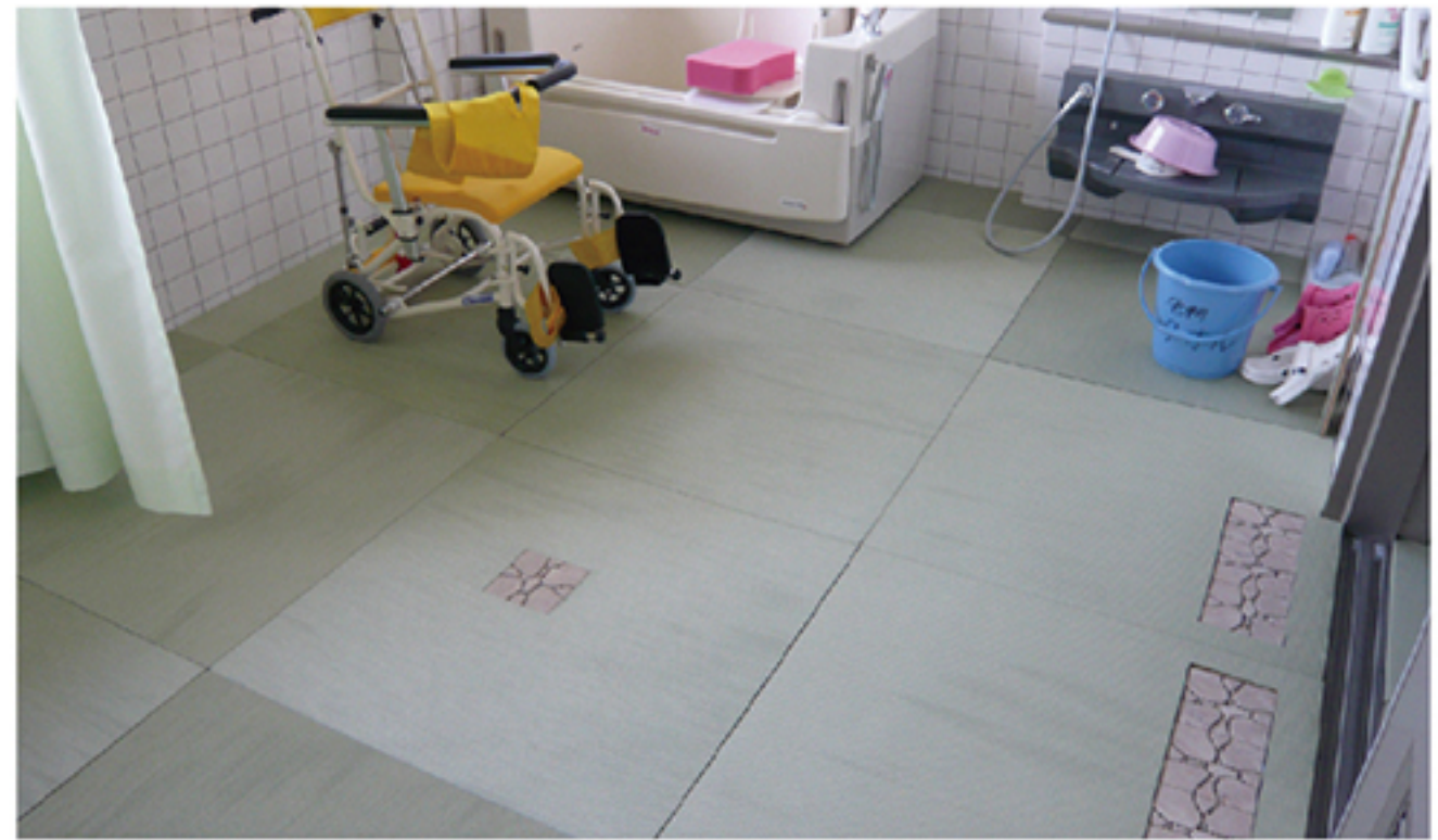
Bathroom at a day care facility (Bathroom Tatami)
