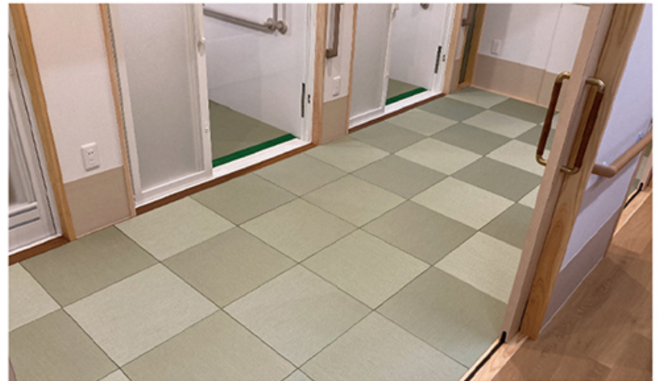
Changing room at a day care facility (Fireproof and washable Tile Tatami)
